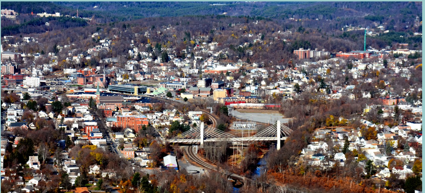
Aerial photo of Fitchburg, MA. (Source: Nick Allen on Wikimedia Commons )
