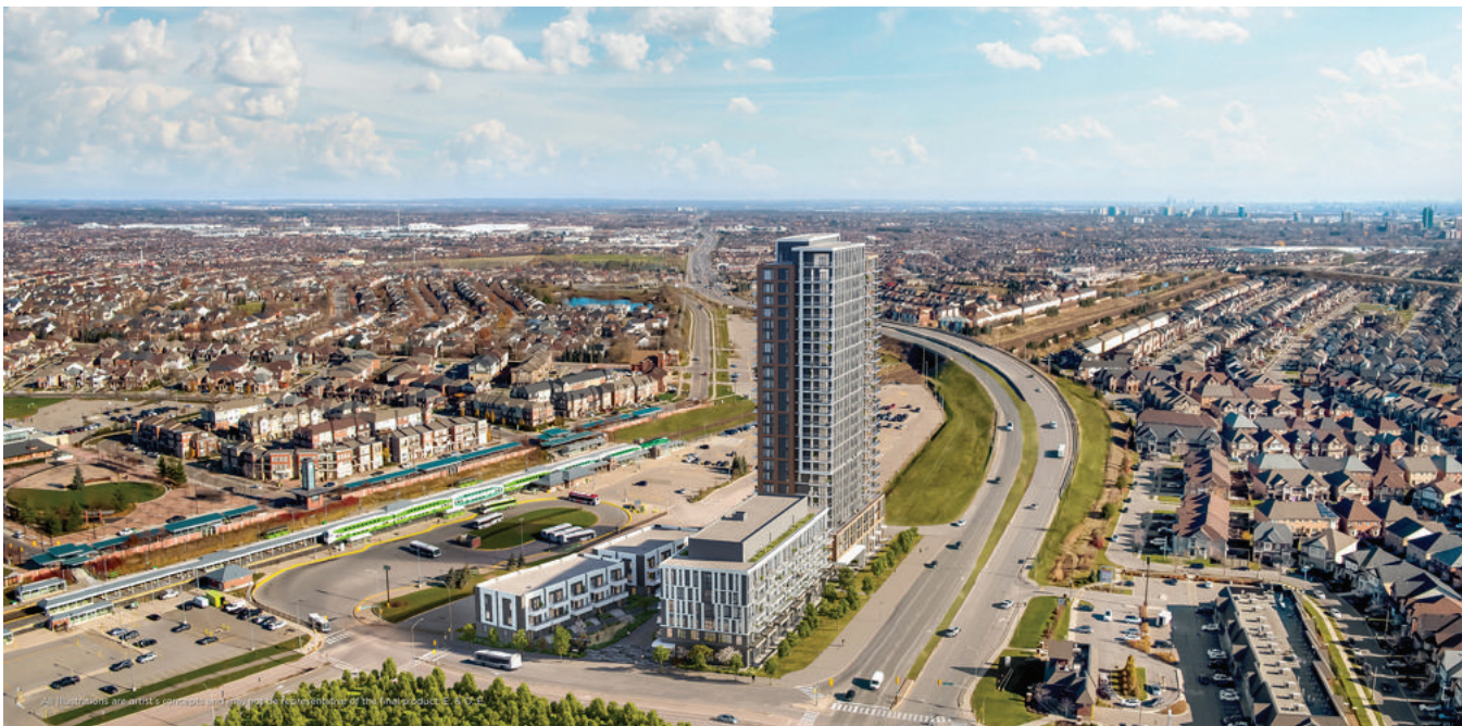
Mount Pleasant Village and associated transit-oriented development. Photo: The Daniels Corp
