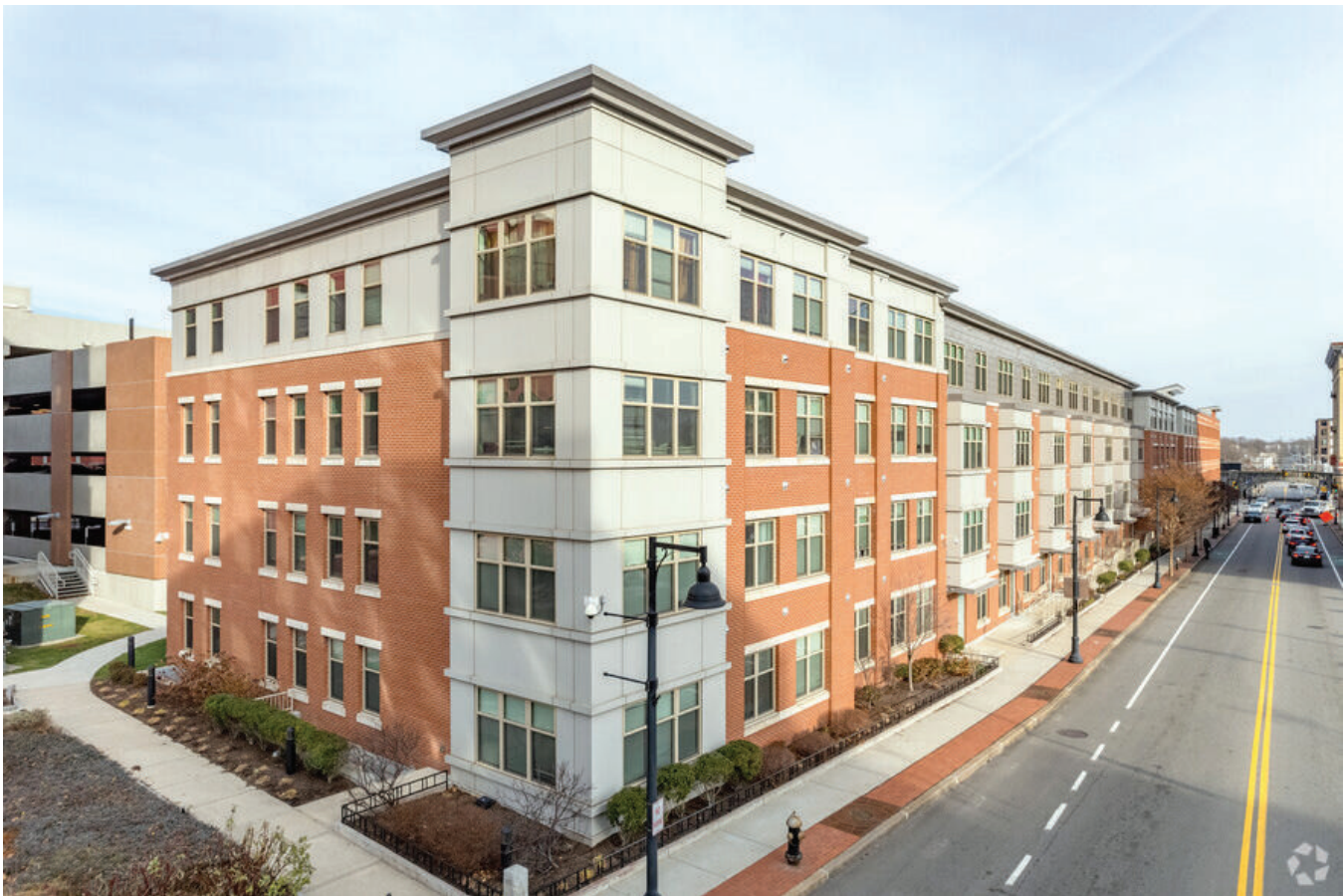
Located across from Brockton Station, Enso Flats is one of only a few recently completed developments in Brockton. Photo: LoopNet
